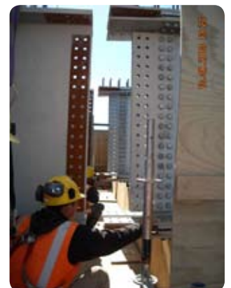
A pair of beams are about to be bolted together.
