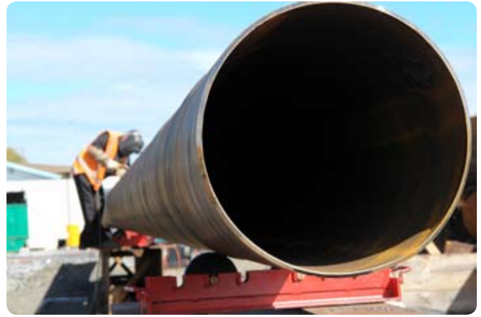
Pile casings measuring 24m and 36m are constructed on site.
