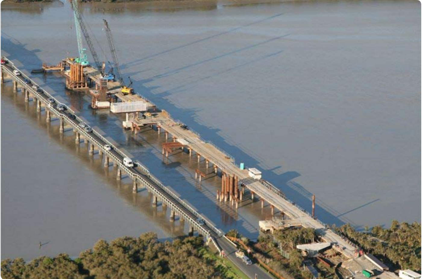
This aerial photo shows progress to June 2010.
