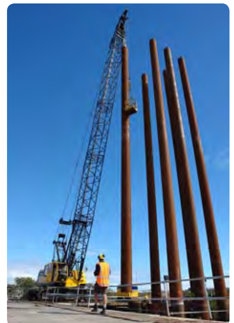
Pile casings being driven beneath the Waihou River
