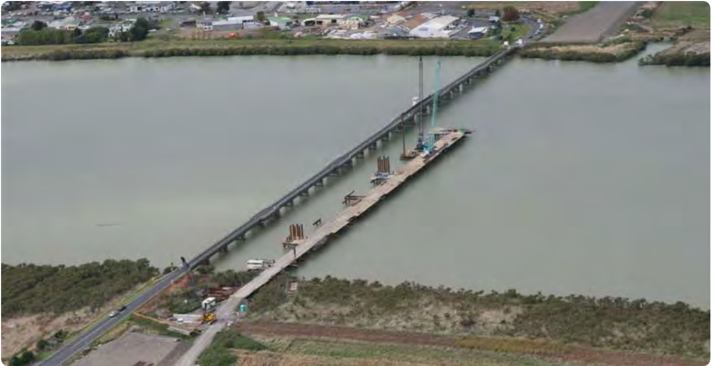
Kopu Bridge progress 7 May 2010
