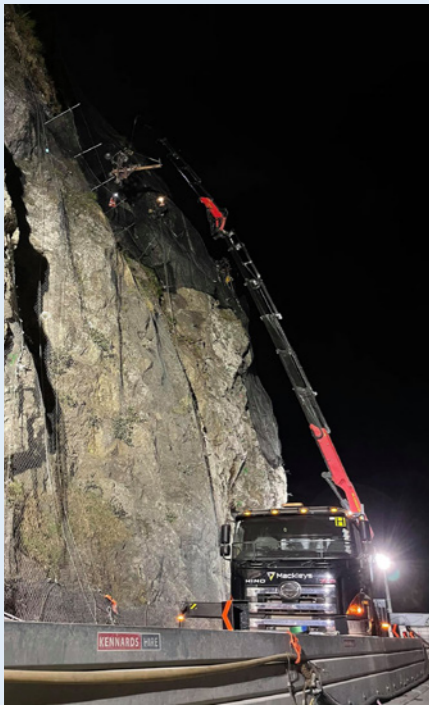
Drilling spot bolts at the very start of the project
