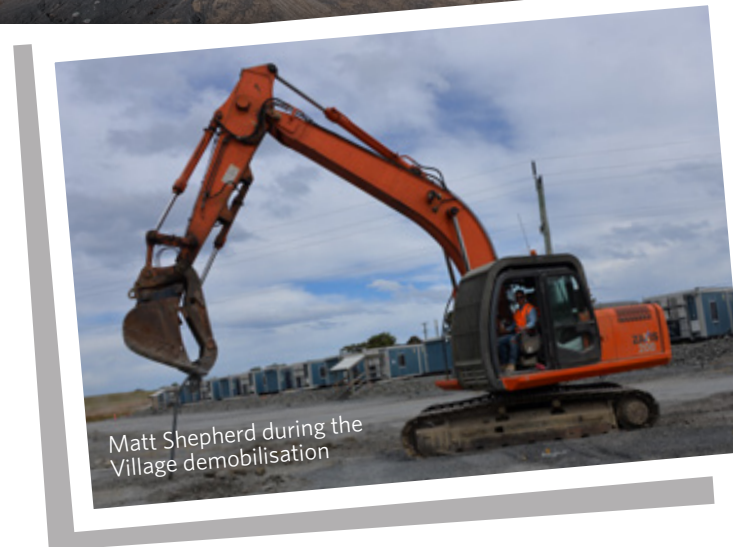
With all units removed, the land reinstatement is now underway at the former NCTIR Village site
