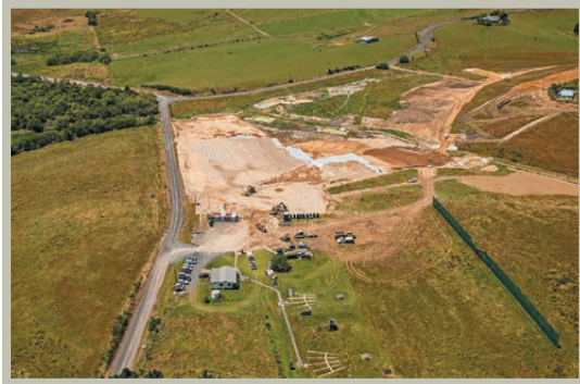
Works to the south of McVie Road
