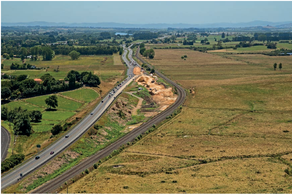
Huntly Northern Interchange works looking north
