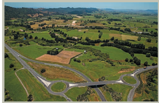
Gordonton Interchange looking north
