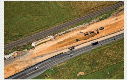
Works at the Huntly Northern Interchange
