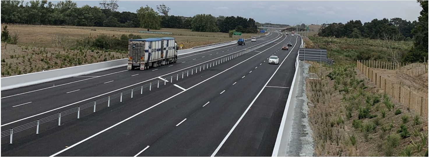
Vehicles on the new section of expressway just south of Waring Road, with the Gordonton Road interchange in the distance.
