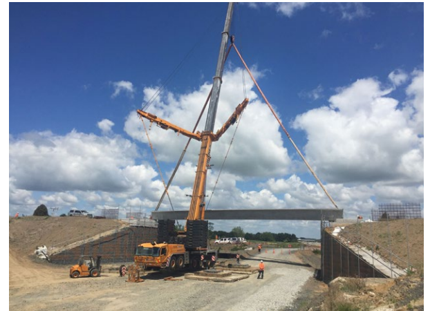
Beams going up on the Waring Road bridge at the southern end of the project.
