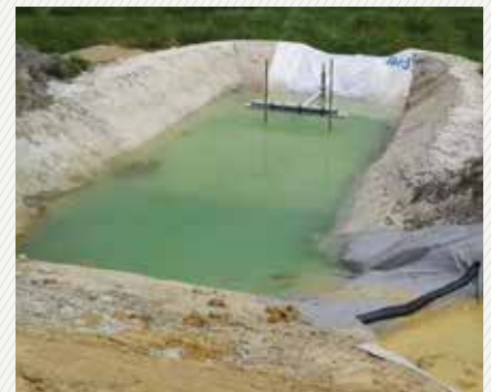
A decanting earth bund.
