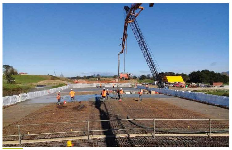
The big deck pour on the Whangamaire Stream bridge required 95 trucks to bring in 520 cubic metres of concrete.
