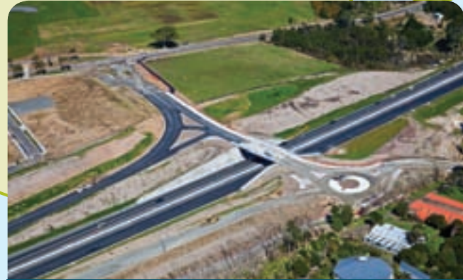
The Squadron Drive bridge will give access to the new Hobsonville Point development.
