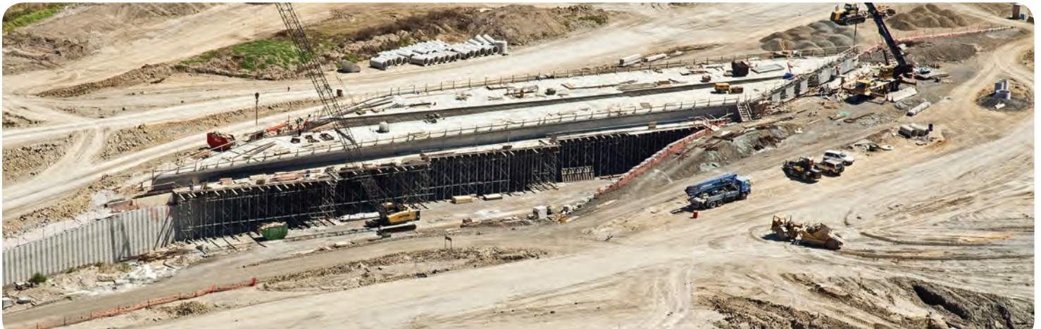
The birdcage supported the flyover as it was being constructed.
