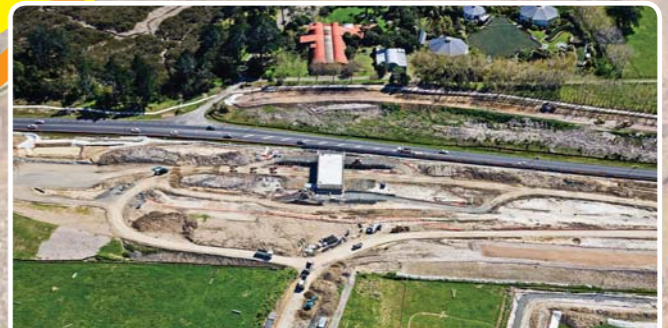
The new Squadron Drive Interchange under construction near Monterey Park
