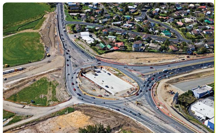
Work continues inside the roundabout at Hobsonville Road
