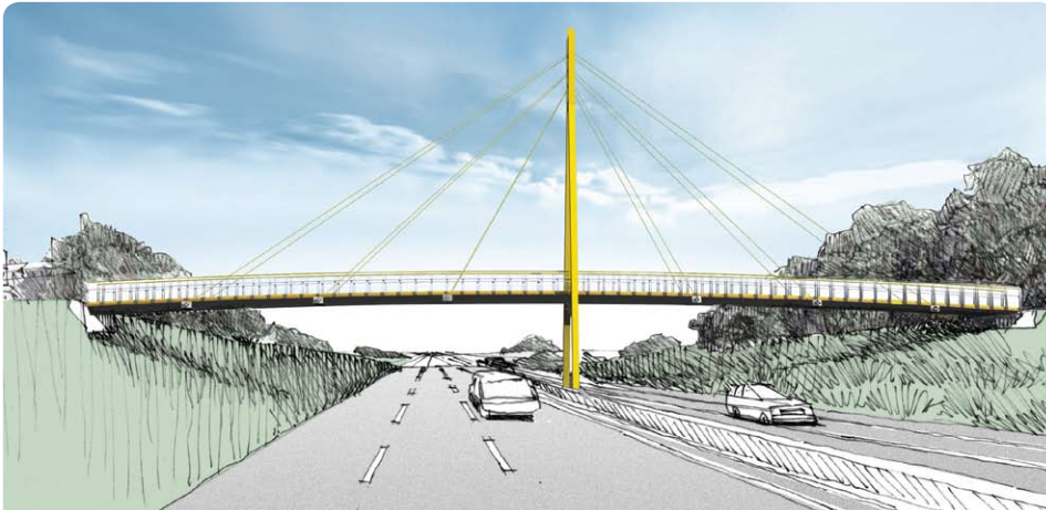
CLARKS LANE BRIDGE a two metre wide cable-stay footbridge for pedestrians and cyclists will give access over the motorway.
