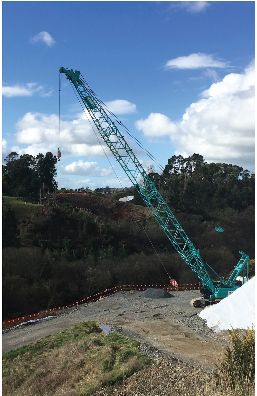
Piling crane in place ready to start
