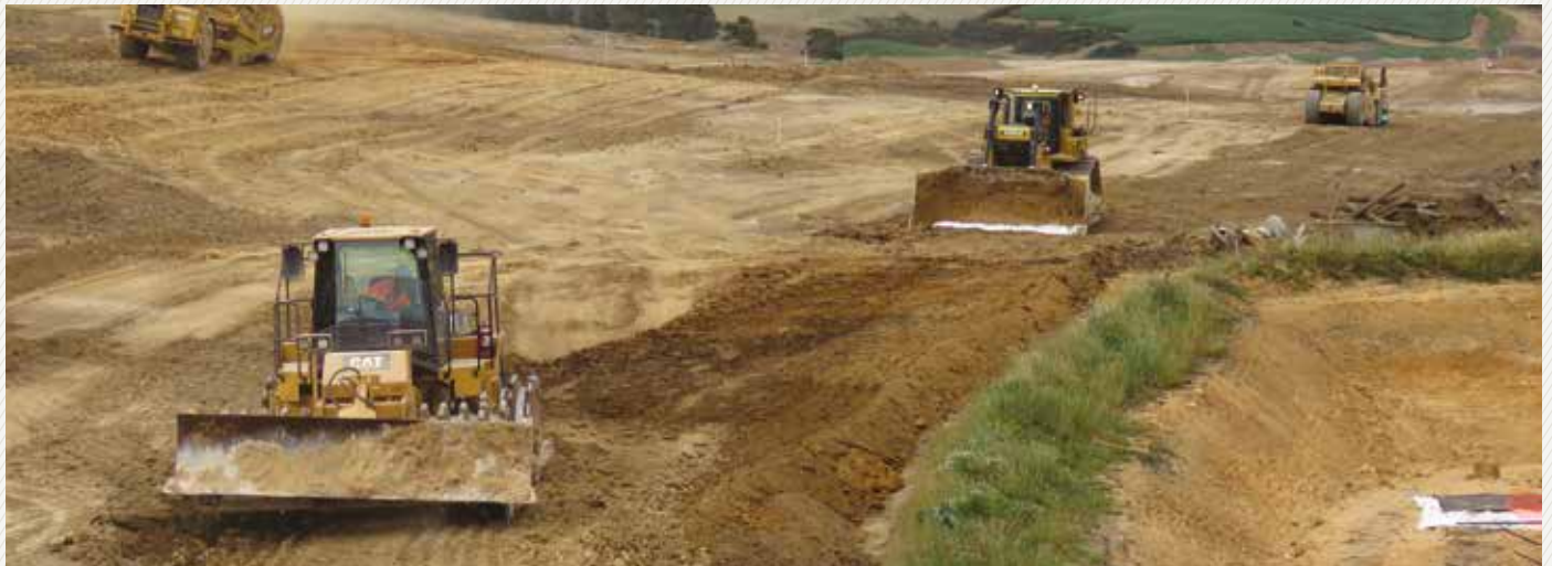
Bulldozers and zv form the expressway embankments near Osborne Road
