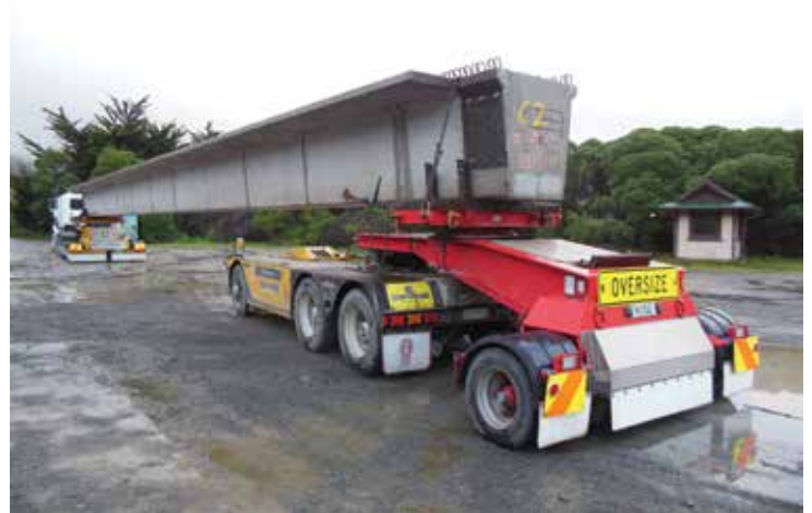
The jinker steers the rear of the beam with its motor turned off, then drives back to base to be loaded with the next beam
