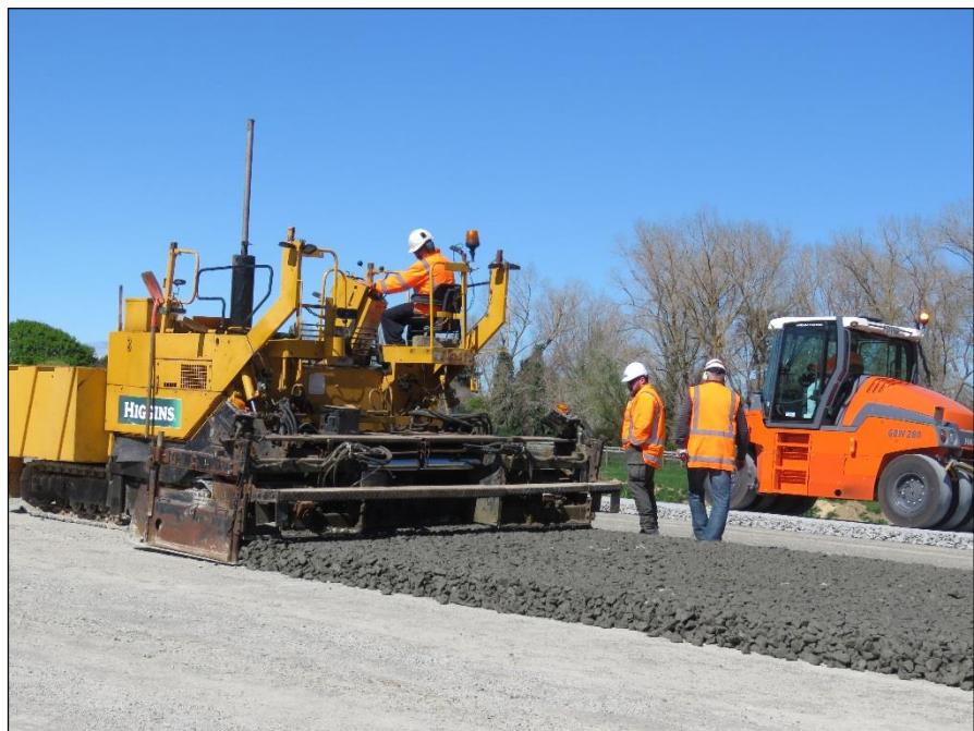
Hi-Lab pavement testing at the Southern Interchange.
