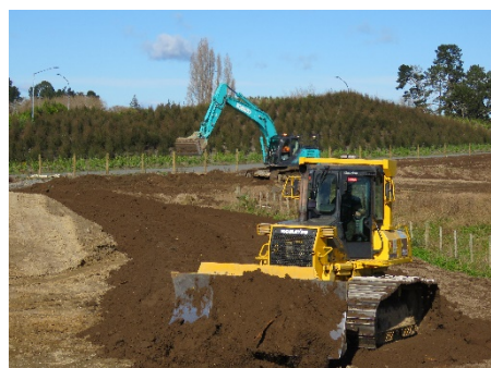
Earthworks under way at the cultural reserve.
