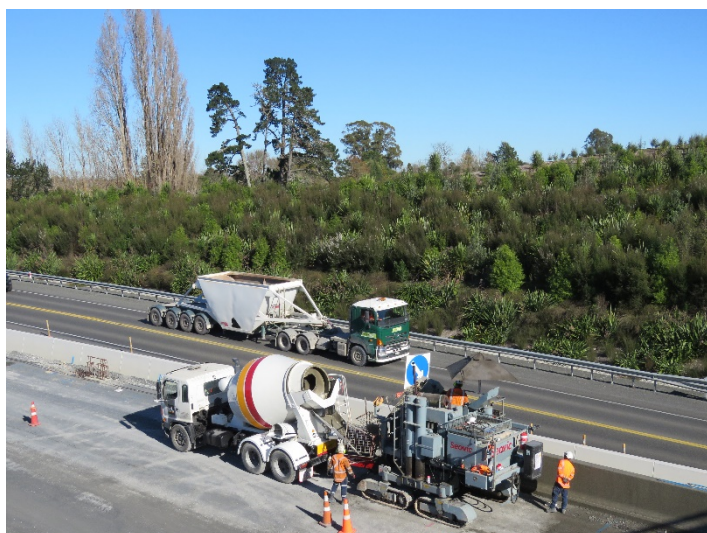
Concrete barriers being formed at the Southern Interchange.
