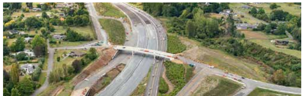
Work continues on local road connections at the Southern Interchange.
