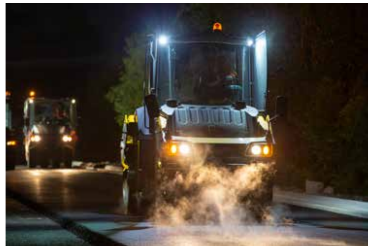
Vibrating rollers compact the asphalt.
