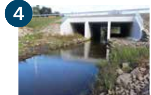
The Kaitemako culvert has environmental benefits to the area
