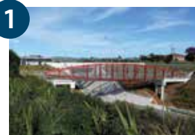
The pedestrian overbridge was built in one piece
