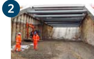
The underpass was built using top-down construction
