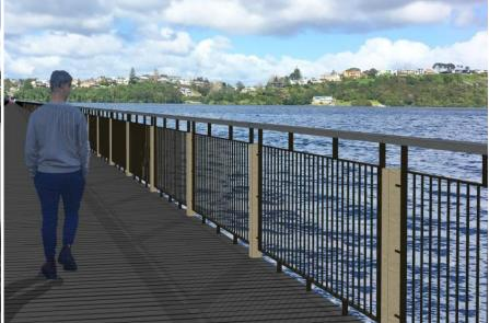
▼ **Style 2:** This style consists of a timber top railing, metal posts and a metal infill. A gap will be created beneath the top railing to further allow 'see through'.
