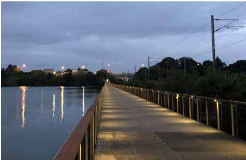
▲ Similar lighting on the completed Section 3 Ōrākei Basin Boardwalk
