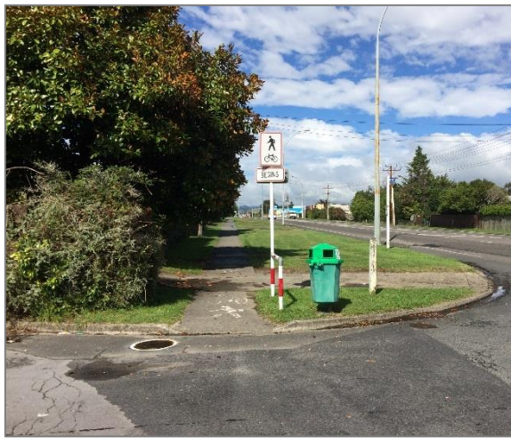
Figure 7-9: Shared path crosses numerous driveways close to property boundaries
