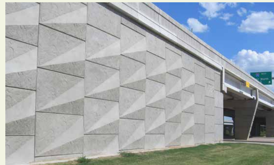
Southern Motorway, Christchurch - pattern of light and shade visually breaks up large walls.
