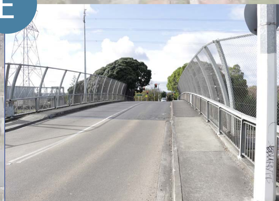
PRINCES STREET BRIDGE
