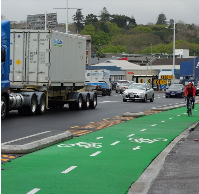
A separated cycle lane on Beach Road, a busy route to the Port of Auckland that's used by 20,000 vehicles a day, compared to about 15,000 a day on the Dunedin one-way system.
