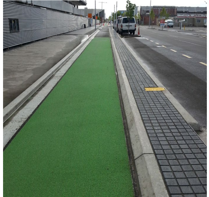
Parking on some sections of the Dunedin one-way system separated cycle lane could be similar to this section of the Tuam Street separated cycleway in Christchurch.
