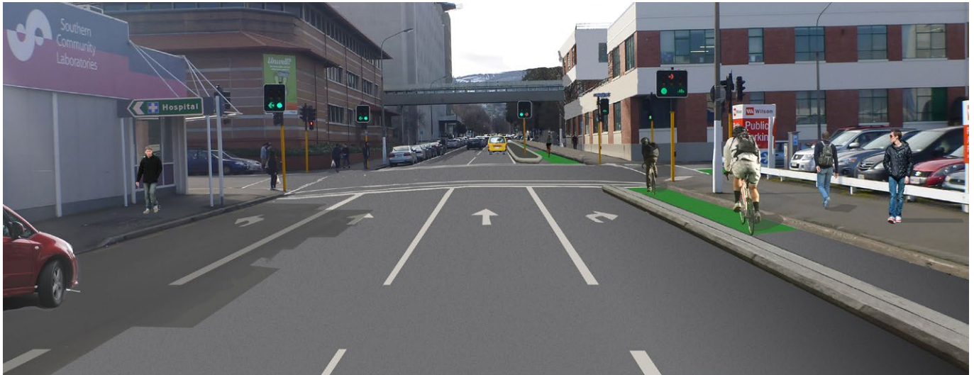
A computer-generated image showing how cyclists and vehicles might be kept apart on the Dunedin one-way separated cycle lanes.
