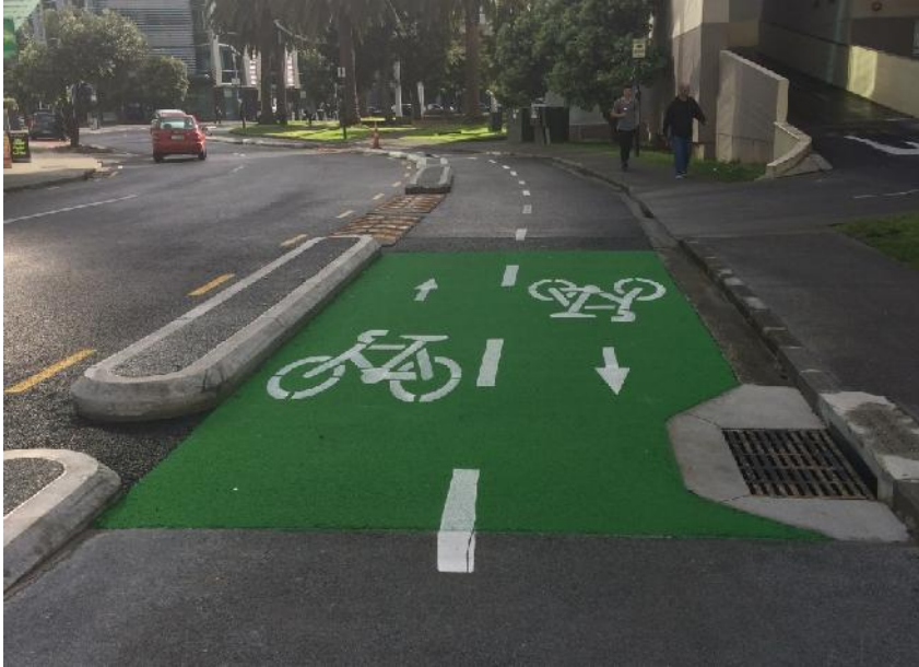
Figure 5-5: Example of cycling friendly sump grate
