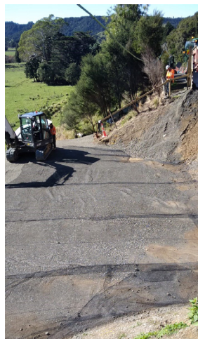
Above: Work underway on retaining wall north of Hicks Bay.
