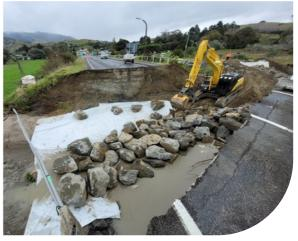
Mangahauini Bridge: The Tokomaru Bay to Te Puia Springs section of SH35 was most significantly impacted by the weather, with the Mangahauini River causing substantial erosion and dropouts, and washing a Mangahauini Bridge abutment away, leaving a 16-metre-wide gap in the highway and cutting access to communities north of Tokomaru Bay.
