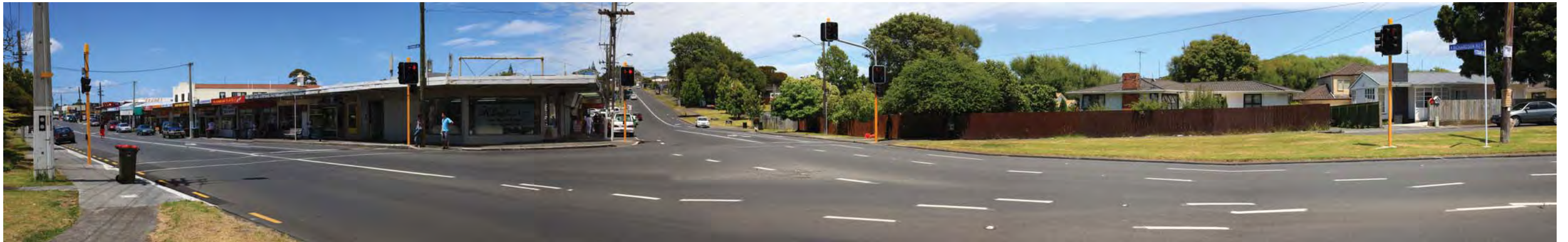
Figure C-9.8: Photo 9-8 Existing Stoddard Road shopping centre looking up Richardson Road towards proposed bridge
