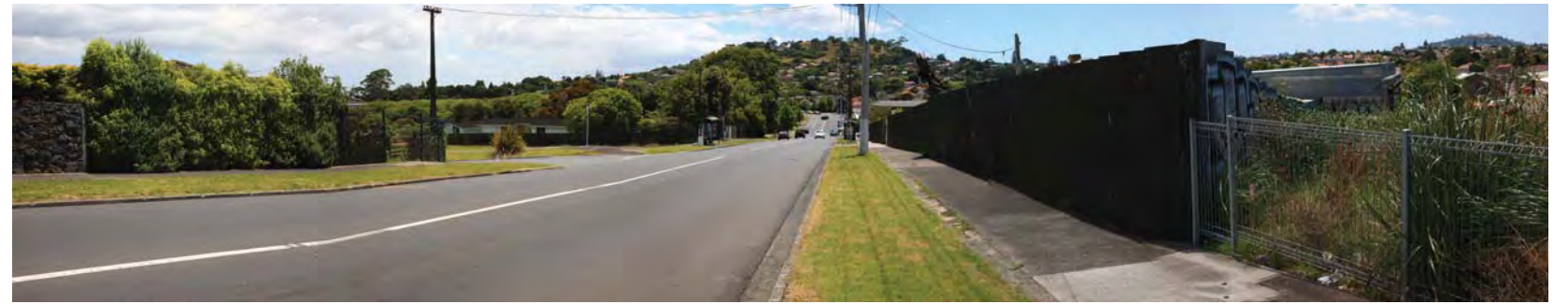
Figure C-9.7: Photo 9-7 View down Richardson Road towards Stoddard Road shops (proposed Richardson Road bridge location)
