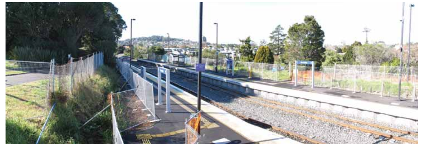
Figure C-8.14: Photo 8-6 The western rail line looking towards Mt Albert Pak n Save
