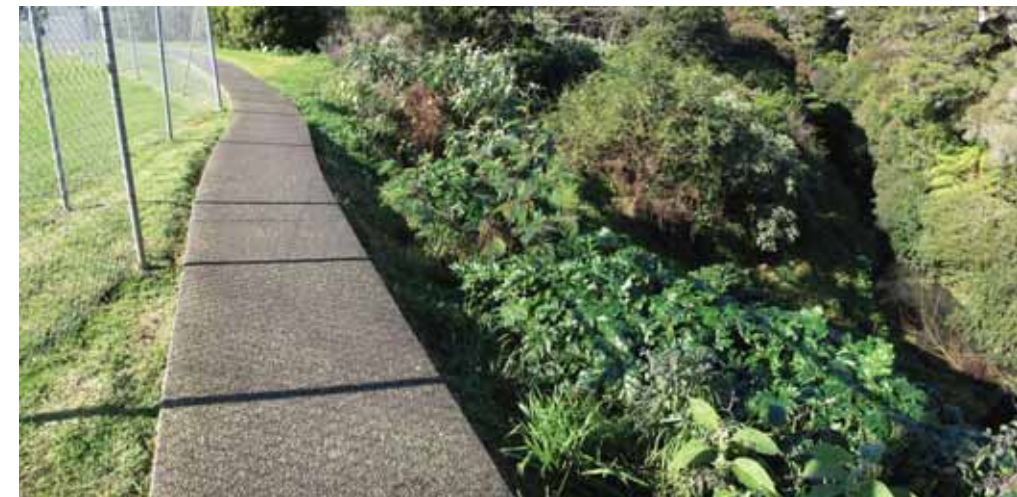
Figure C-8.4: Photo 8-4 The existing pathway network through Phyllis Reserve is narrow and suffering from erosion in places
