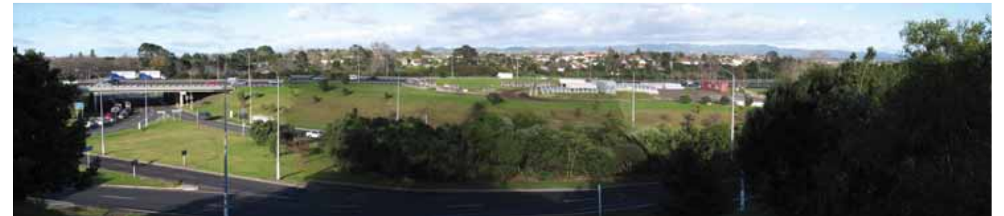
Figure C-5.4: Photo 5-3 Elevated view of Great North Road interchange from Alberta Street
