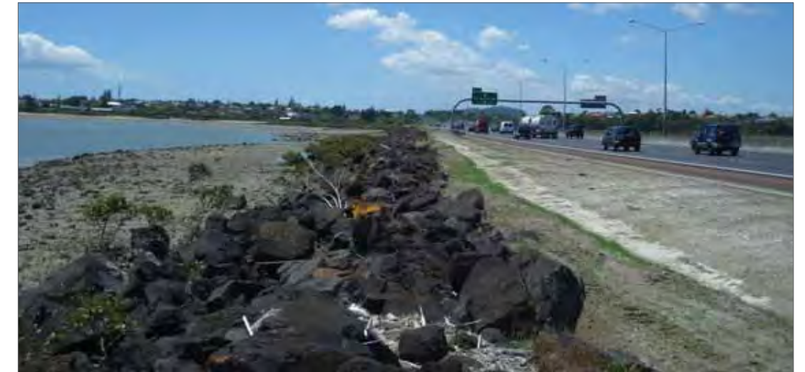
Figure C-4.7: Photo 4-3 Existing view eastwards approaching Rosebank bridge
