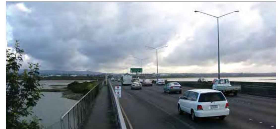
Figure C-4.15: Photo 4-7 Existing view west on Rosebank bridge
