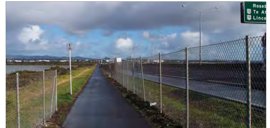
Figure C-4.8: Photo 4-4 Existing view westwards after Rosebank bridge on the off-road route
