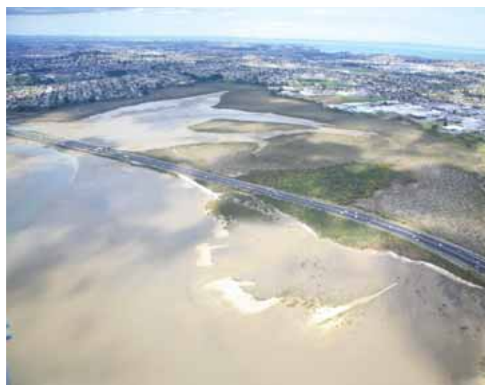
Figure C-4.2: Aerial view of sector 4 from the north
