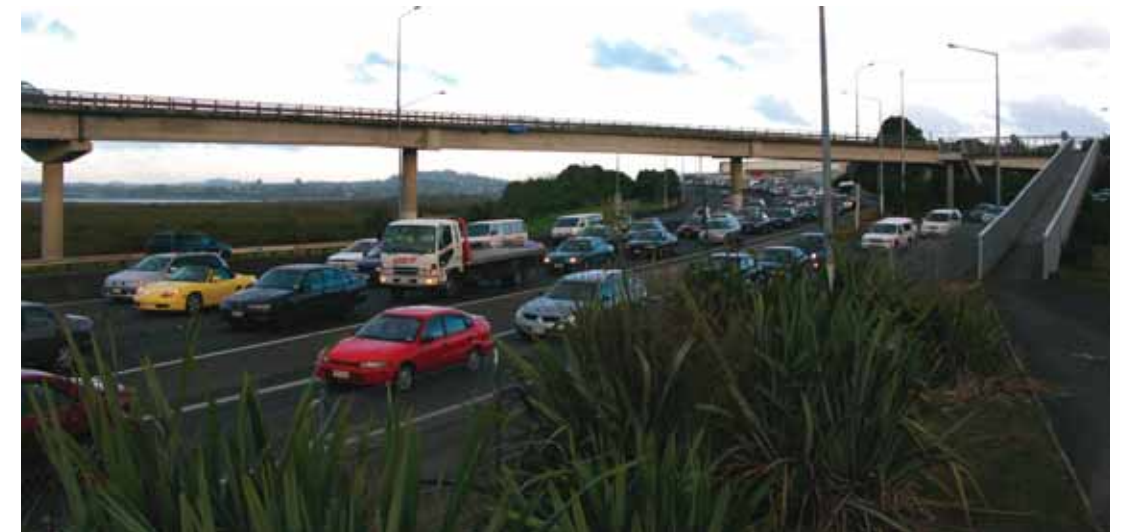
Figure C-3.4: Photo 3-1 Existing view eastwards approaching Patiki overbridge on off-road route
