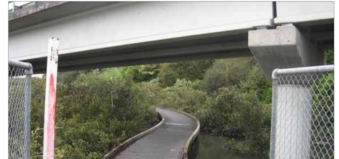
Figure C-3.9: Photo 3-4 Existing cycleway boardwalk underneath Rosebank off-ramp
