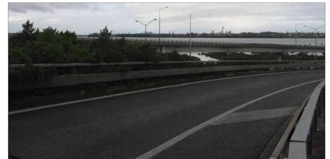
Figure C-3.11: Photo 3-6 Existing view westbound, between Rosebank ramps
