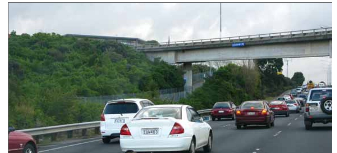
Figure C-3.10: Photo 3-5 Existing view westbound, between Rosebank ramps
