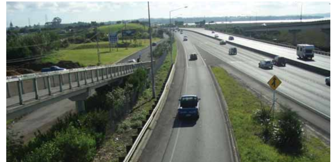
Figure C-3.3: Photo 3-2 Existing view westwards from Patiki Photo
