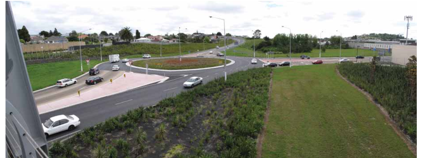
Figure C-10.79: Photo 10-8 View from pedestrian overbridge west towards the proposed interchange
