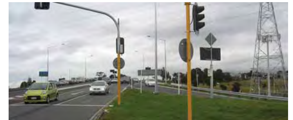
Figure C-1.19: Photo 1-5 Existing view south of overbridge and cloverleaf ramp
