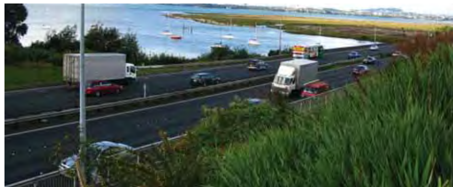
Figure C-1.15: Photo 1-1 Existing view east, located west and south of the Whau River
