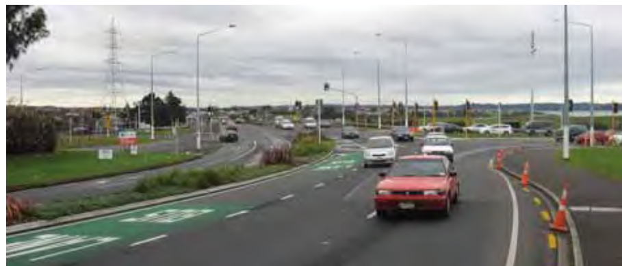
Figure C-1.17: Photo 1-3 View north adjacent to Te Atatu Road, south of the motorway
