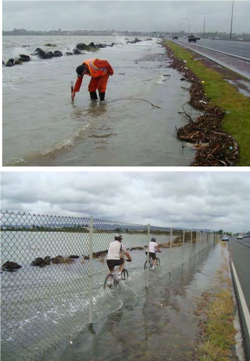
Figure 2.2 – Photographs Showing Inundation (Top: Northern revetment, Bottom: Southern revetment and pedestrian/cycle way)
