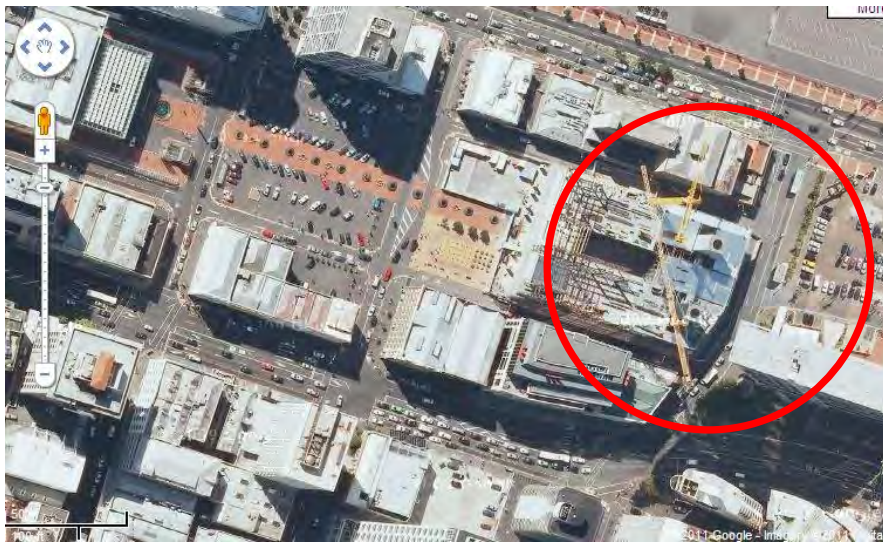
(Above) Stacks in their relocated position above the East Building (under construction).
