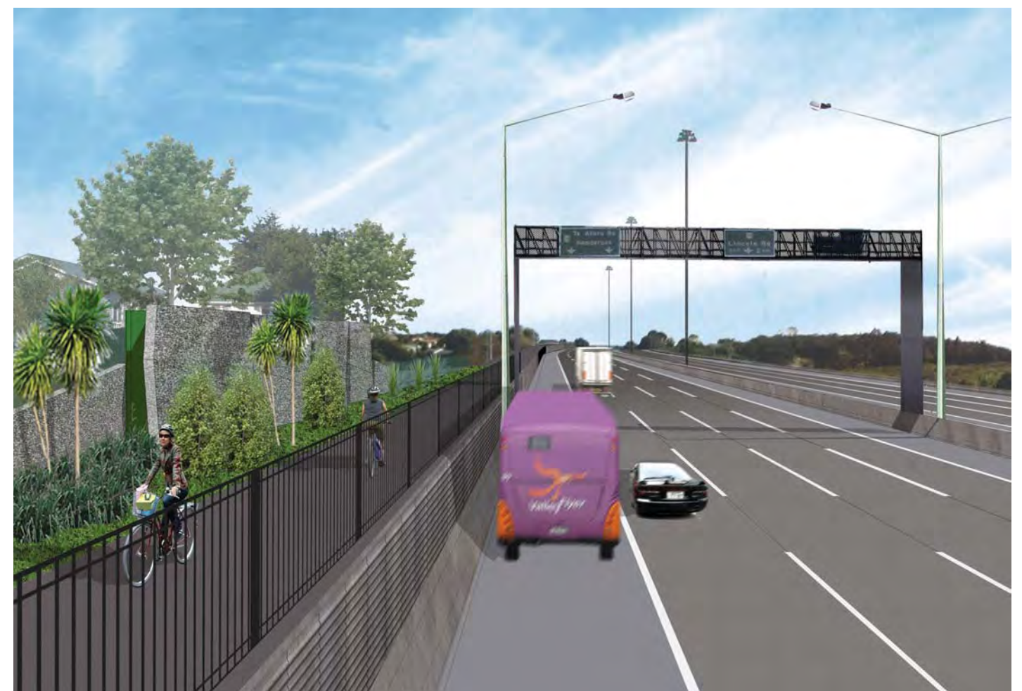
Figure B-26: Artist's impression of retaining wall, fence, noise walls, lighting and signage gantry – SH16
