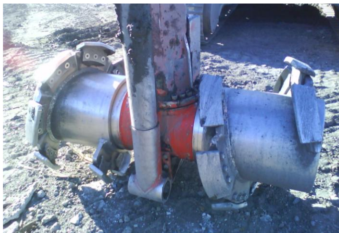
Figure 1.5 - In-situ Mudcrete Mixing Head
