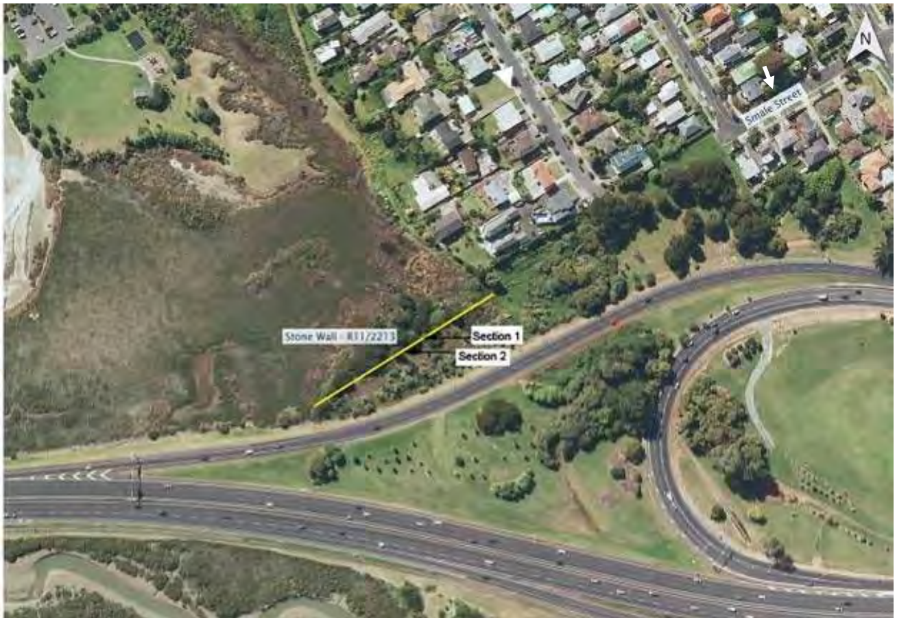
Figure 6.35: Location of stone wall R11/2213, and wall sections surveyed in detail
