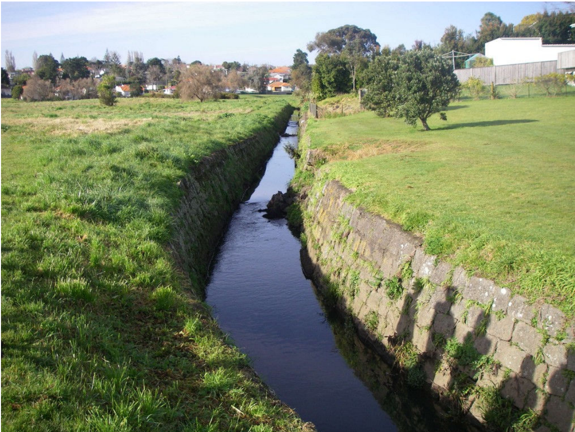
Figure 5.9: Oakley Creek in Alan Wood Reserve showing basalt rock wall channel section
