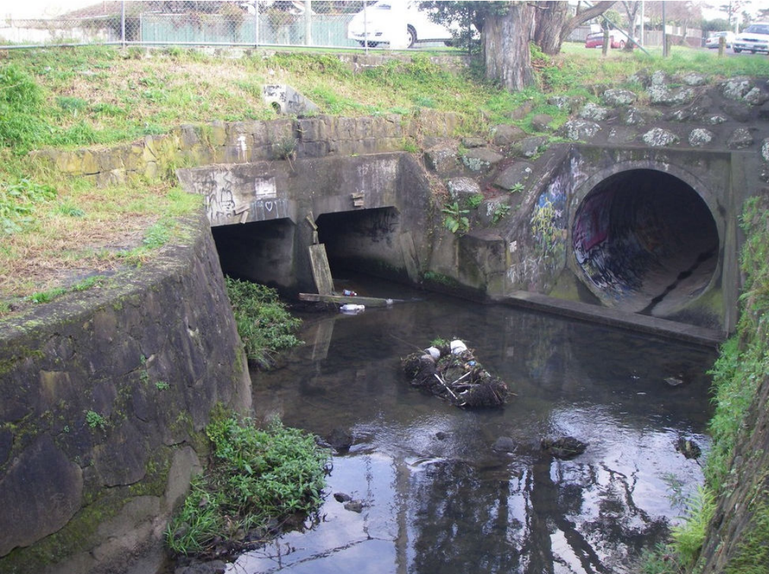
Figure 5.10: Bollard Avenue and Bollard Overflow culvert
