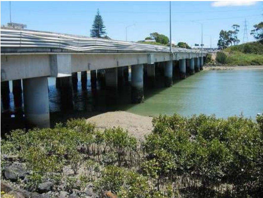
Figure 5.4: Whau River Bridge
