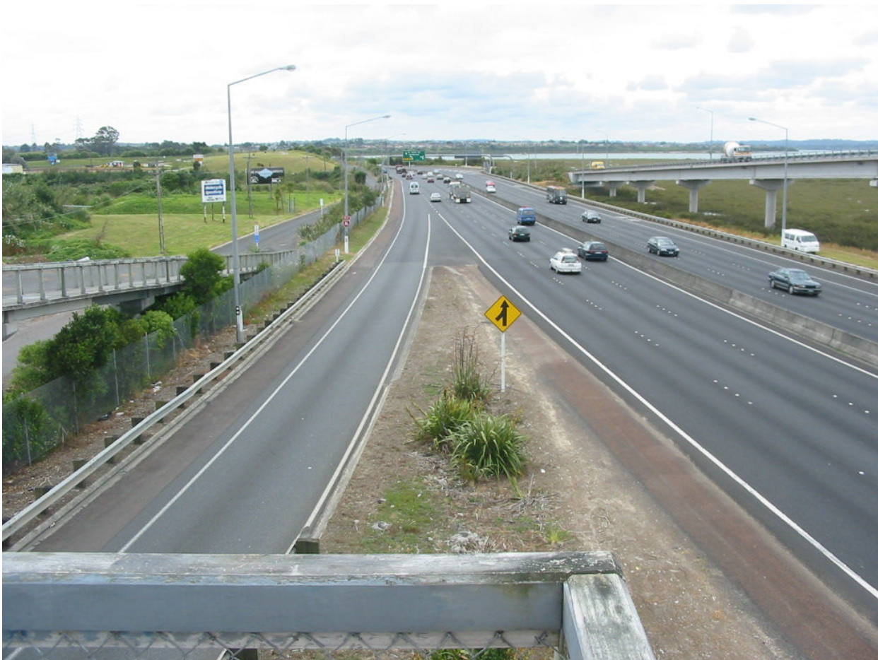
Figure 5.5: Patiki Road onramp looking westward
