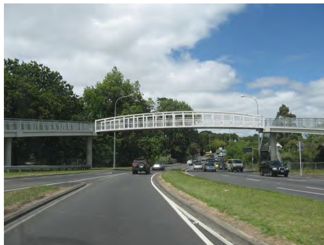
Figure 5-25: Great North Road Overbridge
