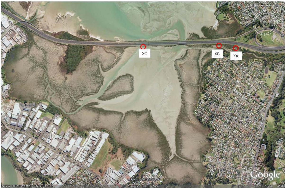
Figure 23: Location of channel re-alignment works (image from Google Earth).
