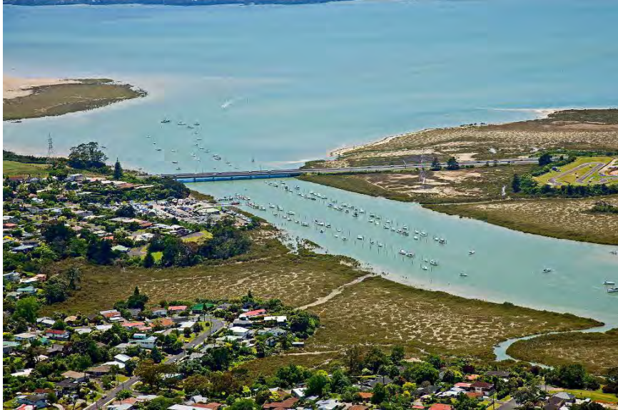
Figure 8.5: Existing Whau River Bridge (Looking North)
