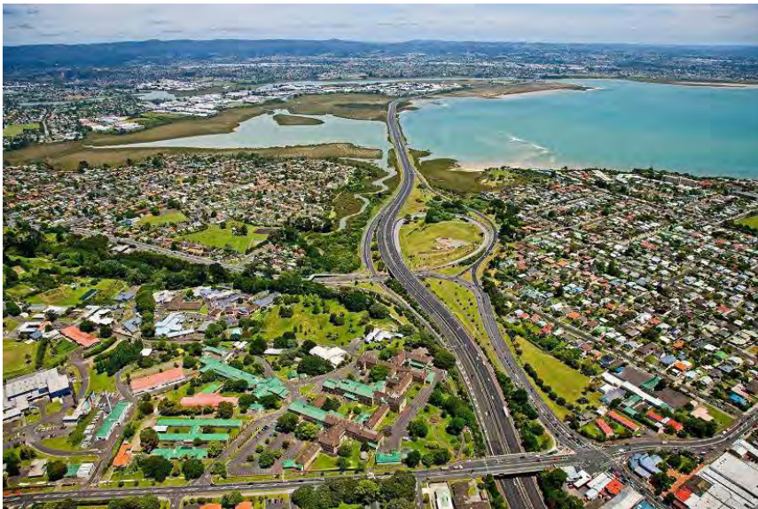
Figure 8.9: Great North Road Interchange (Looking West)
