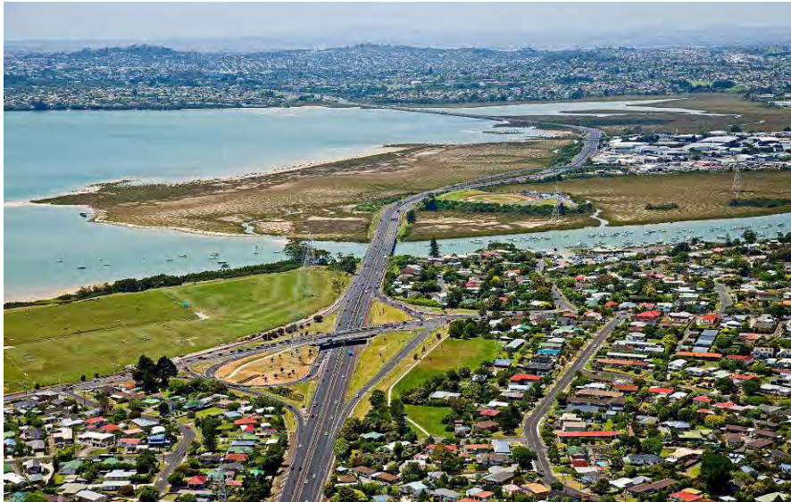
Figure 8.3: Existing Environment - Te Atatu Interchange (Looking East)
