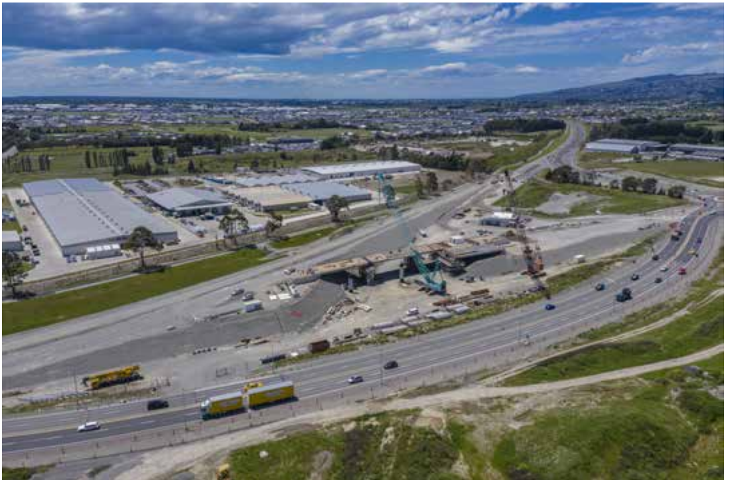
Halswell Junction Road interchange looking towards the city
