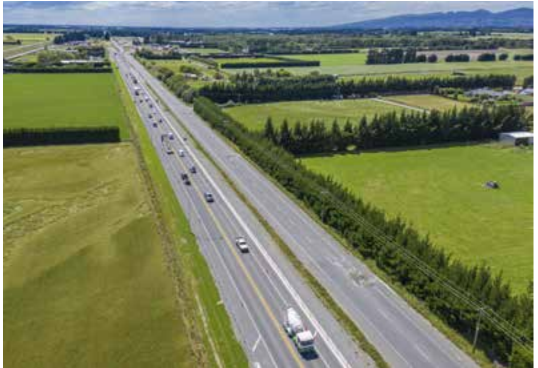
Traffic travelling on the new SH1 northbound lanes
