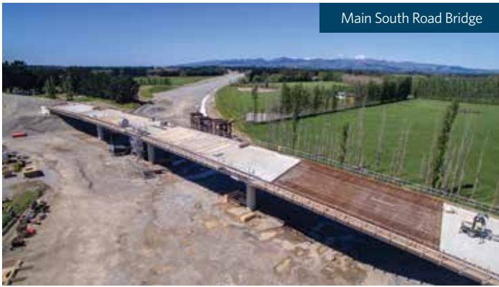
Main South Road beams going into place earlier this year
