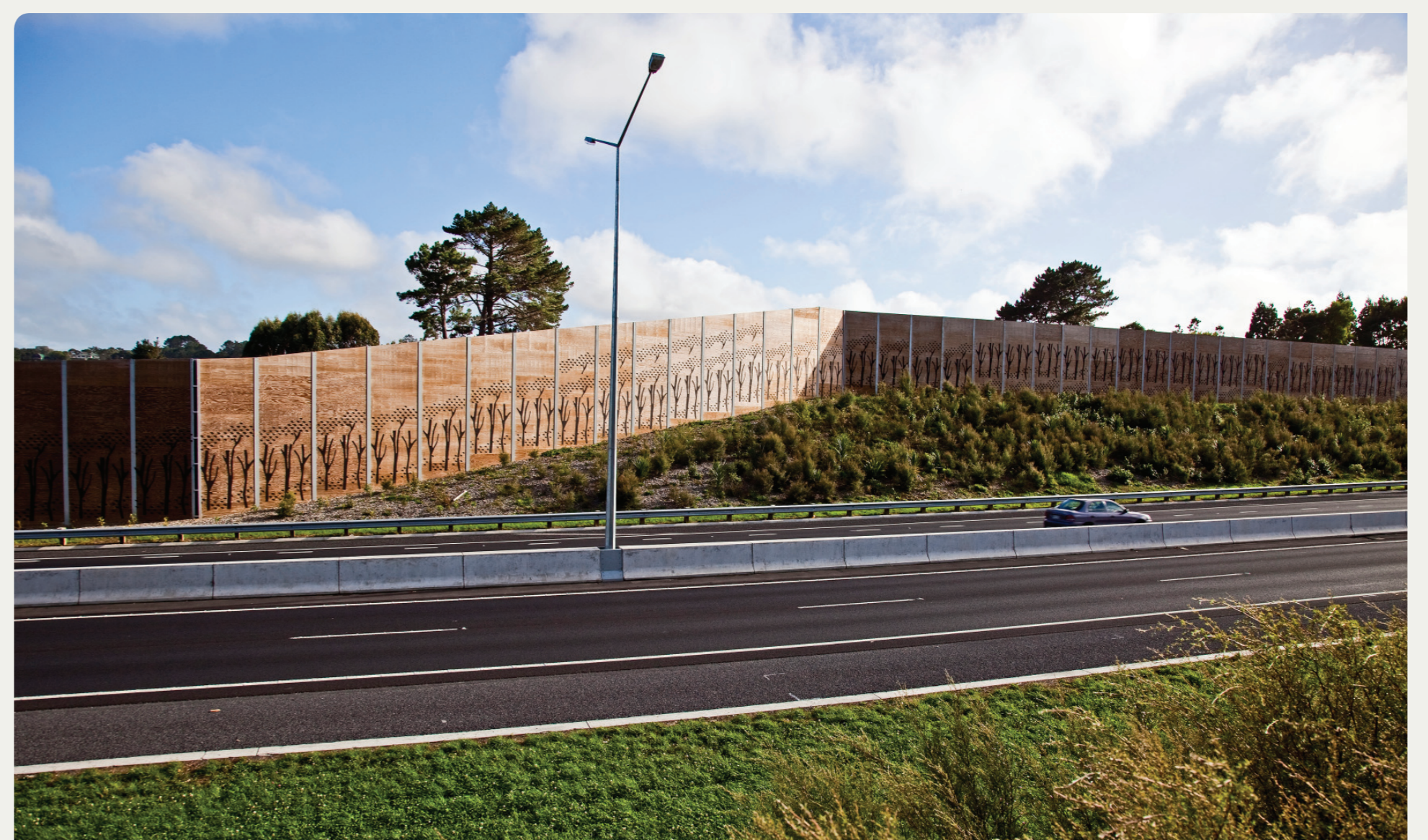
Combined earth bund and noise wall (SH18 Auckland)
