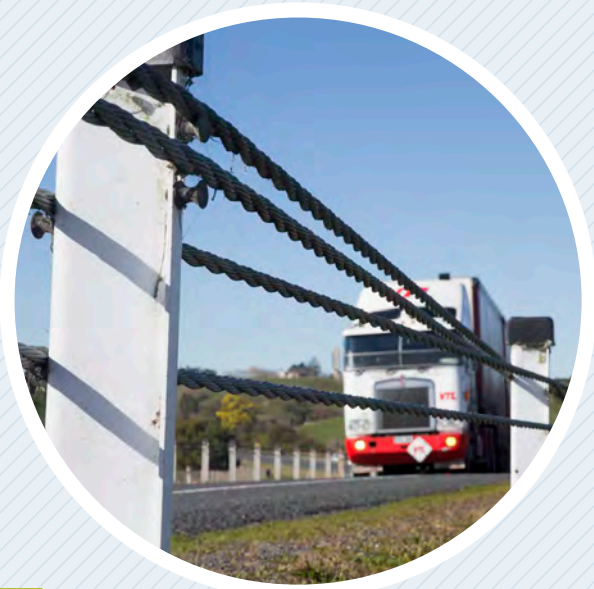
An example of roadside safety barriers
