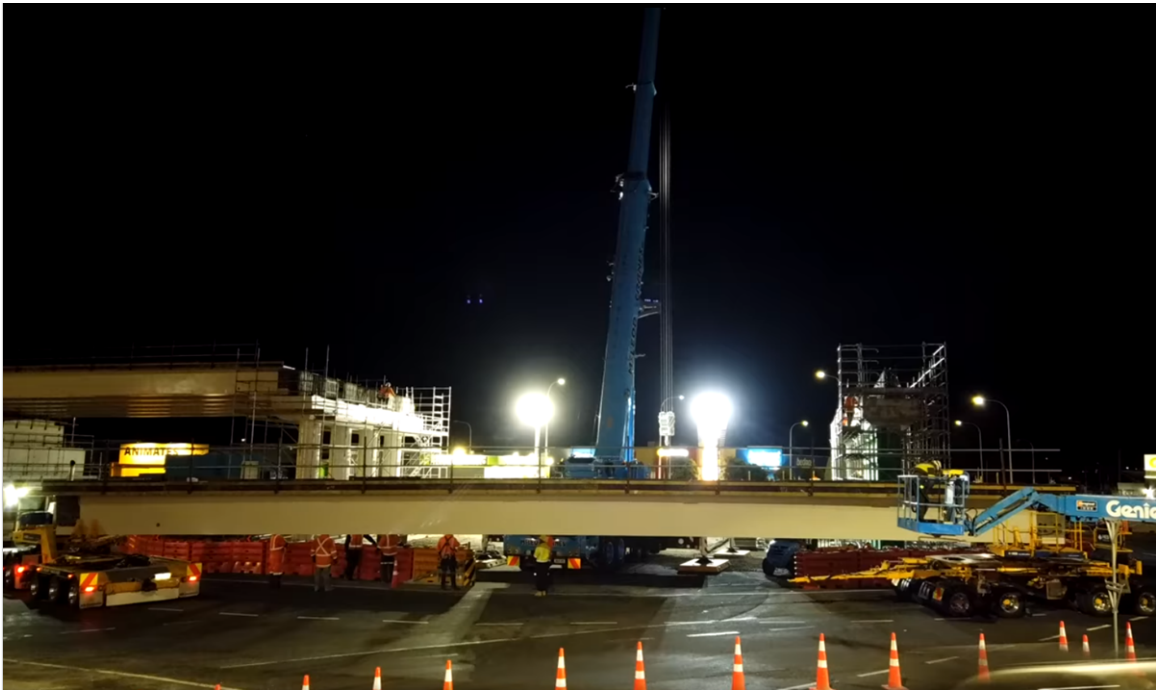
Video: Beam lift timelapse
