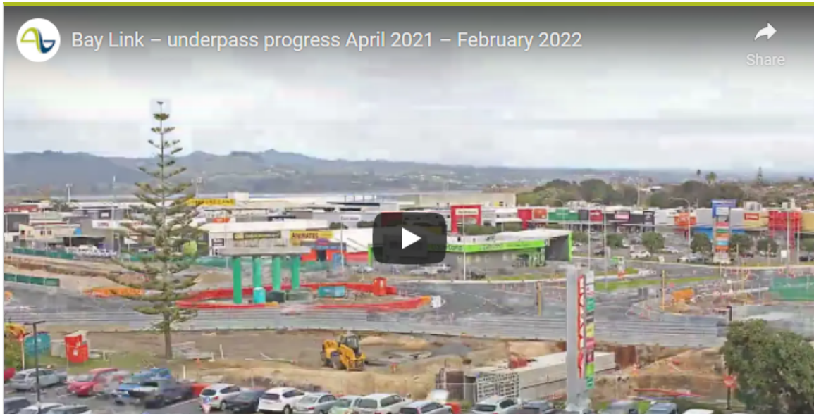
Underpass construction timelapse
