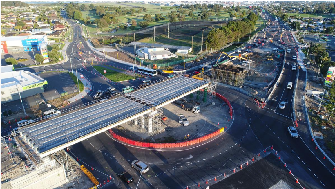
Bayfair roundabout before and after the beam lift
